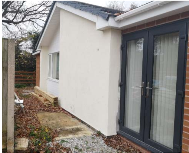
Side elevation of existing bungalow showing main lounge window and patio doors on extension facing new dwelling.
